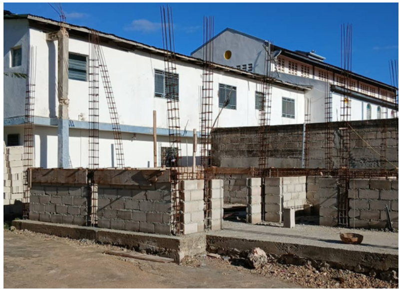
Progress on the classroom at the Professional Center
