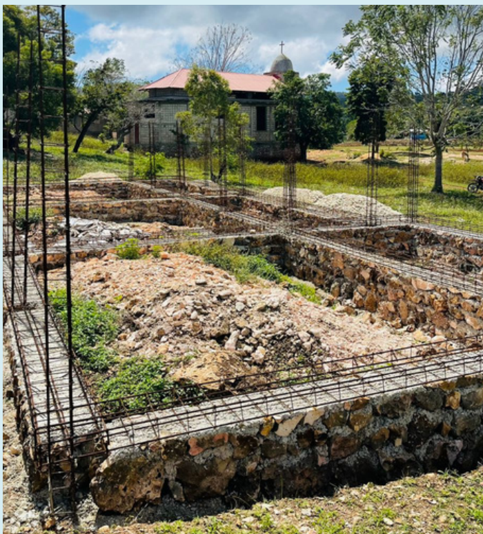
Les Saints Innocents classroom foundation is laid!
