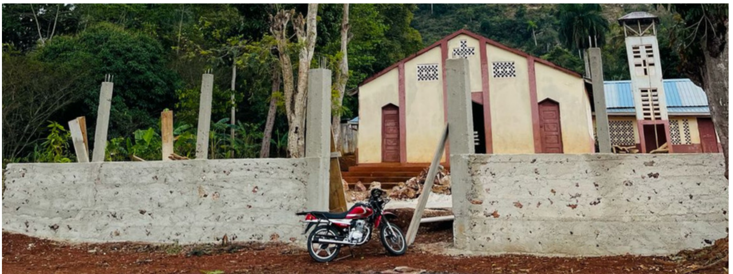
Front entrance at St Jean Baptiste where a gate will be installed
