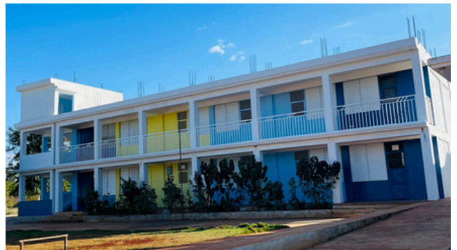
The middle/high school building has 6 classrooms
