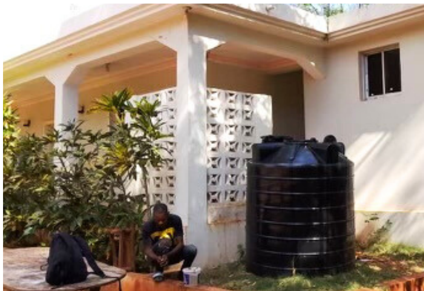
Temporary cistern next to the kitchen & bath
