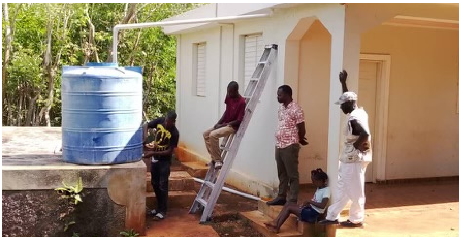
This groups tests a second tank installed on top of an old cistern in Lotoré
