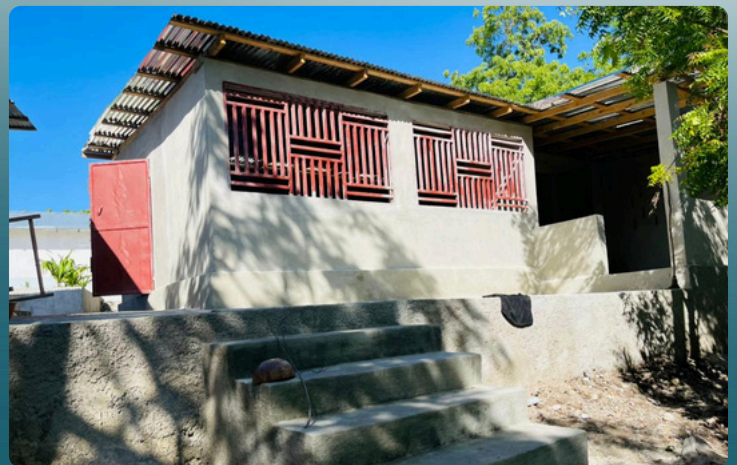
New kitchen in Bois Brûlé
